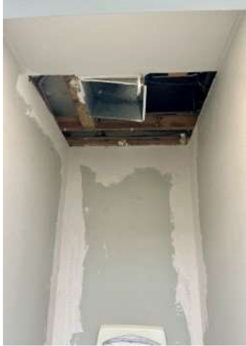
Another view of the bathroom in Bldg. 1
